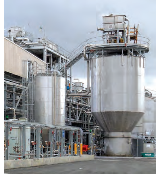
Australian Paper's wastepaper recycling and de-inking plant in Victoria.
